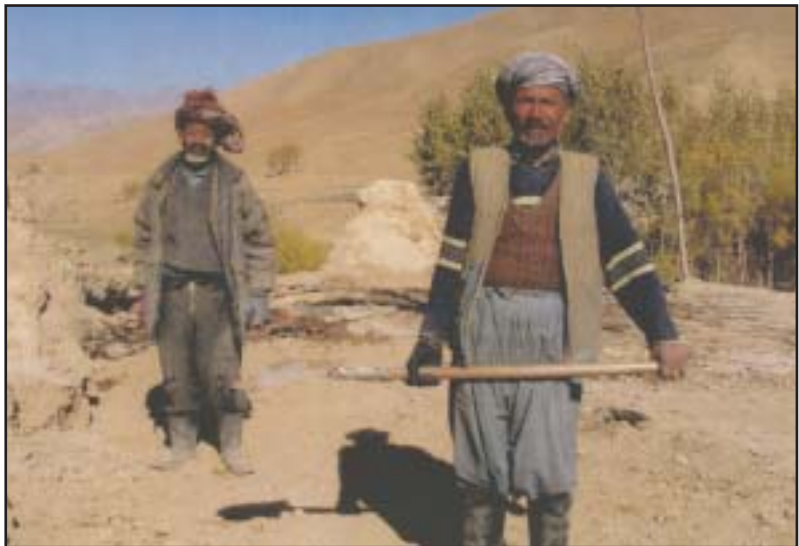
Top & middle: Rebuilding houses in Shah Qadam, Shibar District, Bamyan Province
