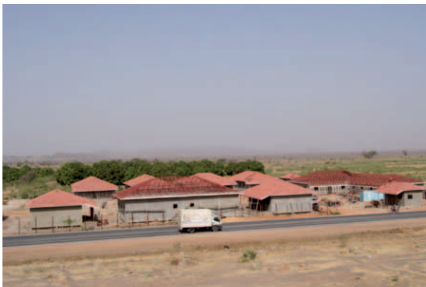
Civil Service Training Centre in Kadugli, Southern Kordofan, nearing completion, February 2011. Photo: UNDP.
