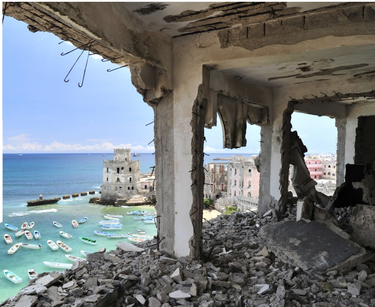
Mogadishu's luxury hotel the Al-Uruba lays in ruins after two decades of civil war. Though building work in Mogadishu is on the rise, it may still be several years before many of the city's buildings will be restored. PHOTO: TOBIN JONES / AU-UN IST PHOTO
